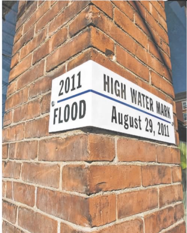
The high water mark from Tropical Storm Irene is seen on Elm Street in Waterbury on Wednesday. GLENN RUSSELL/FREE PRESS
